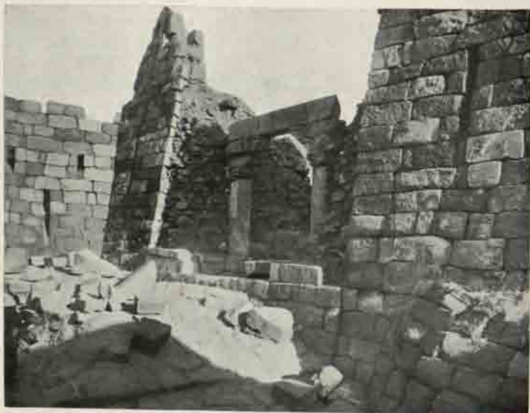
Adilabad west gate, inner entrance before and after excavation.
